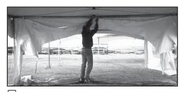
3. Attach clips to Cable: Slide Wall.
