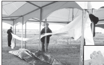
2. Starting with one side, slip joiner underneath tent top flap (B) (see above diagram) and fasten velcro.
