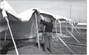
Bases of sidepoles exactly on previously marked positions.
