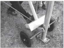
Tighten the ratchet webbing straps. Sidepoles should be vertical upon completion.
